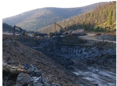
Excavation & Removal of Tailings/Impacted Soils
